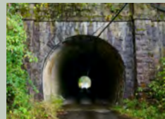
11 Funagaya Tunnel (64 m)
