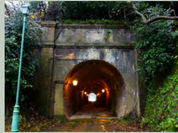
14 Kashimagari Tunnel (87 m)
