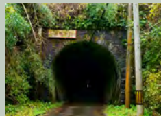
10 Sorojidani Tunnel (401 m)
