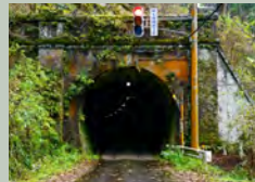
4 Iradani Tunnel (467 m)
