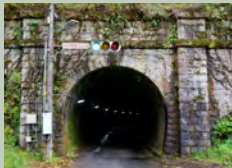
1 Yunoo Tunnel (368 m)
