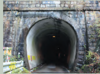
15 Yanagase Tunnel (1352 m)
