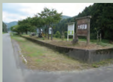
2 Remains of Ogiri Station
