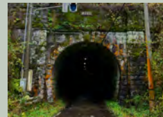
12 Habara Tunnel (979 m)
