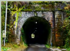
8 No. 1 Kannonji Tunnel (82 m)
